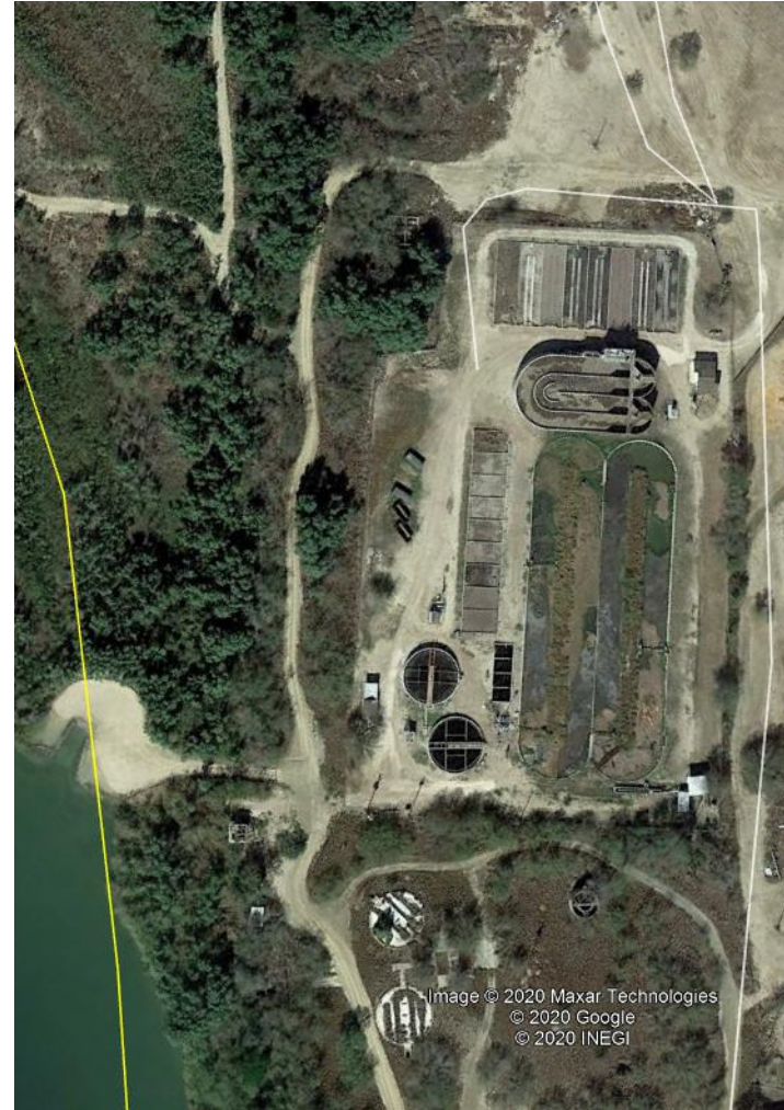
Wastewater Treatment Plant
